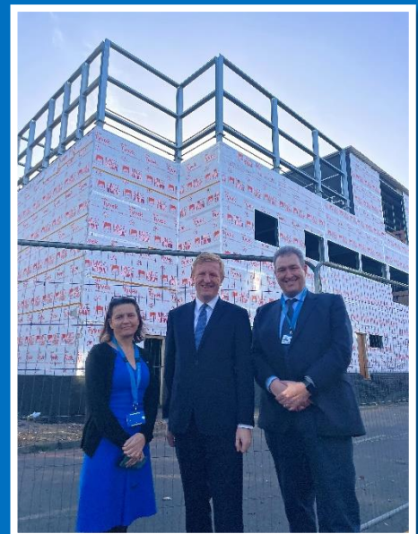
Oliver at the new Watford General Hospital Site
